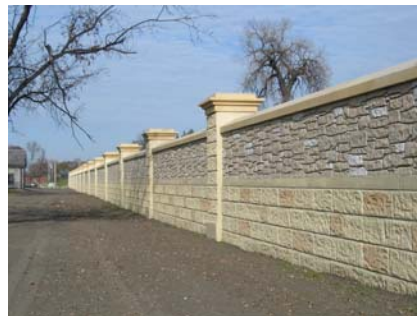
Floodwall at Grand Forks
