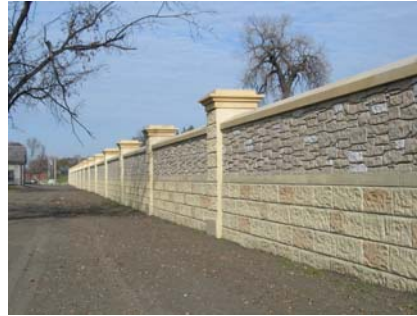
Floodwall at Grand Forks
