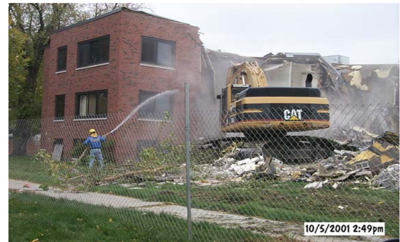
Building Demolition in Grand Forks, ND
