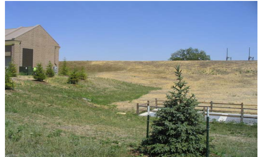
Levee and Pump Station in Grand Forks
