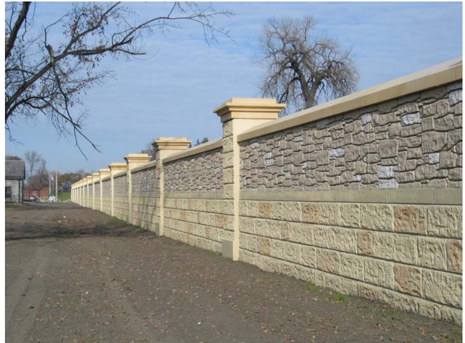
Floodwall at Grand Forks
